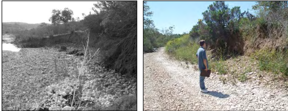
a) Streambank Erosion along Rose Creek above Interstate 805
