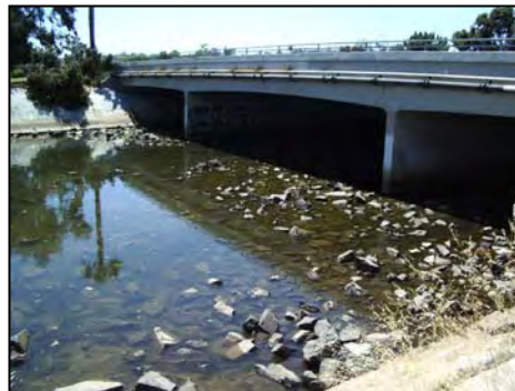
d) Streambank and bed protection below Grand Ave Bridge
