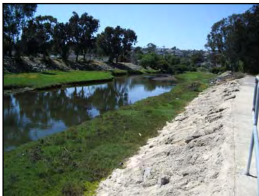
Photo: Figure 5g Date: May 31, 2006 Location: Lower Rose Creek upstream from Grand Ave View: Upstream towards Garnet Ave Flow: Tidal Description: The creek is tidally influenced up to Garnet Ave. This portion of Lower Rose Creek has riprap sides with salt marsh vegetation.
